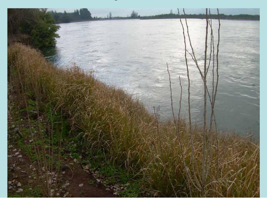
A small section was eroded during the first winter due partly to poor compaction and partly to the poorer growth of the bare root stock.
